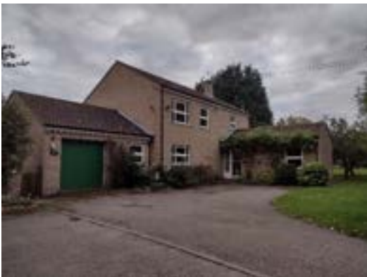
The front of the house taken from the car parking area. The Minister's Study is to the right of the front door and the kitchen window is to the left.
